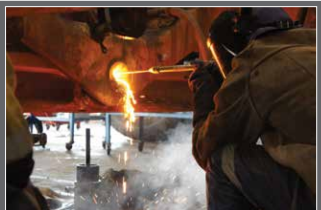
Equipment Workshop Mechanic undertaking hotworks process during a track dozer repair
