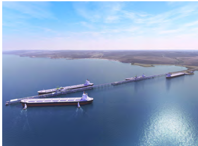
Stage 2 – Cape Hardy port precinct comprises Panamax and Capesize berths and associated infrastructure for bulk commodity minerals, grain and other goods
