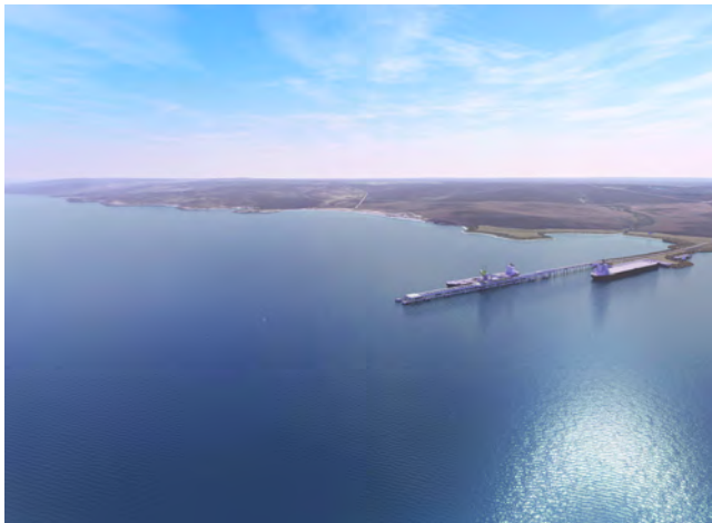
Stage 1 – Cape Hardy port precinct comprises Panamax berth and associated infrastructure for grain and other goods
