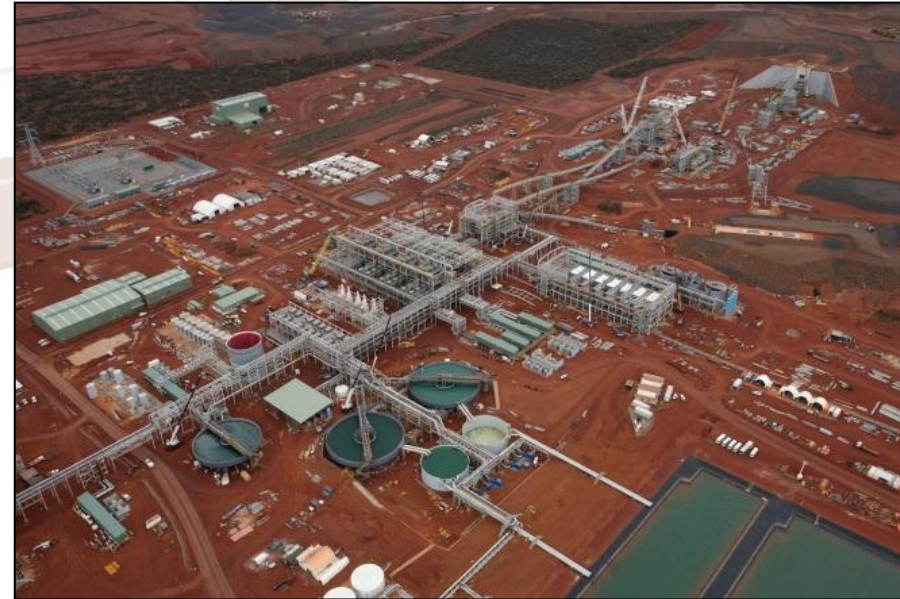
Aerial view of the Karara Iron Project, WA
