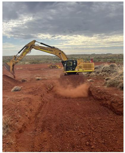
Figure 2: Commencement of Trench Excavation of Detritals
