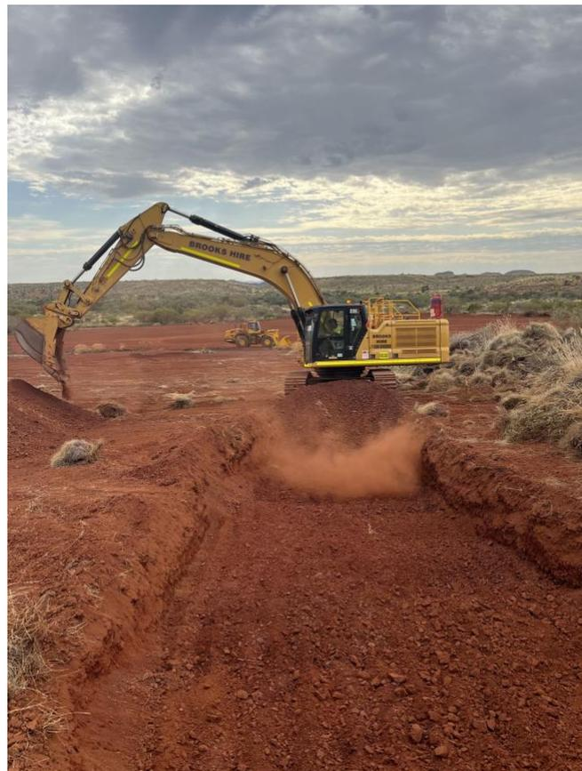
*Figure 7: Commencement of Trench Excavation of Detritals*
