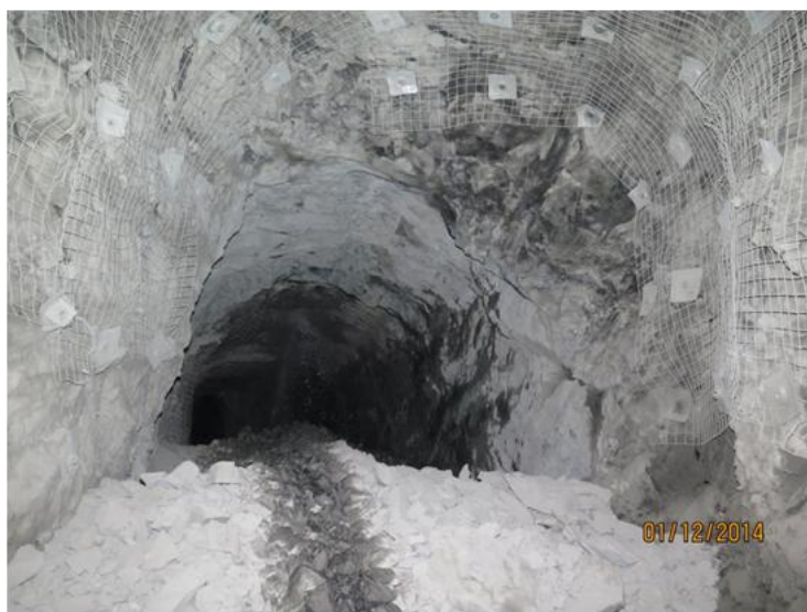
Breakthrough cut of the North Lode incline/decline access taken shortly after firing
