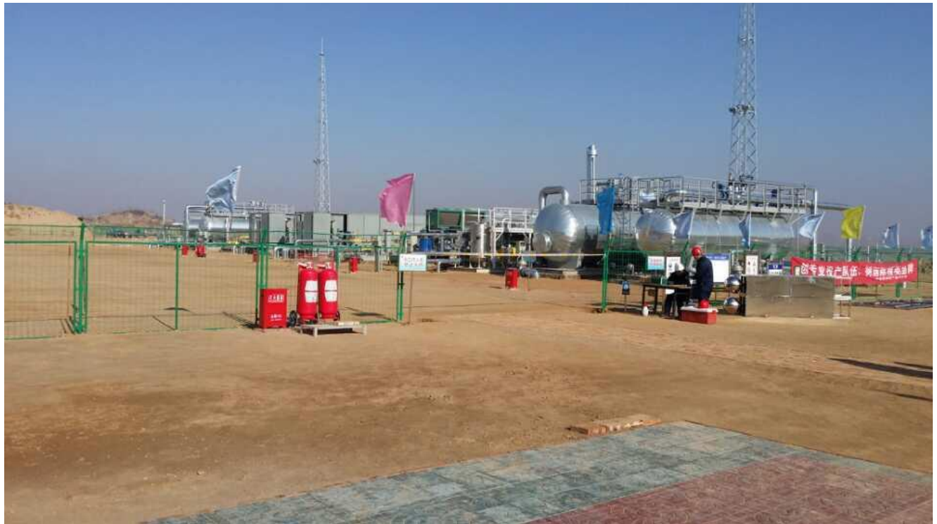
Facilities commissioned at the Sanjiaobei central gathering station
