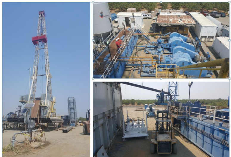
Rig #9 and associated equipment at Dempsey 1-15
