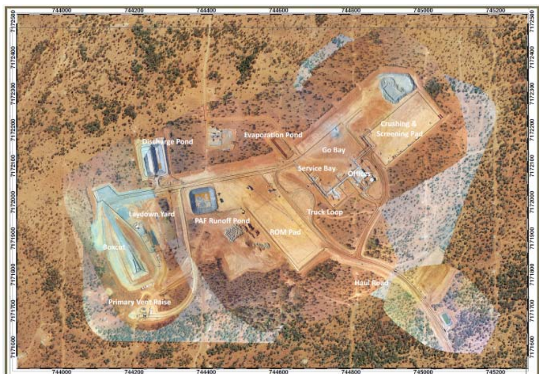
Figure 1: Aerial view of the Monty Project development showing completed infrastructure at Quarter-end.
