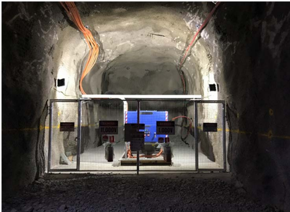
Figure 3: Underground ventilation pumping station, Monty underground mine.
