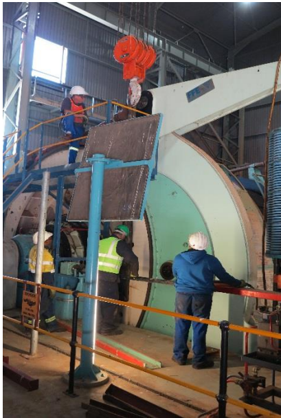
Manually turning the winder – pre dismantling
