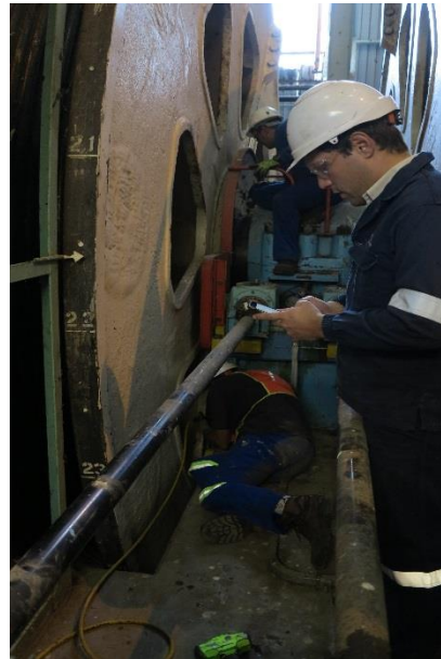
Measuring tolerances – pre dismantling
