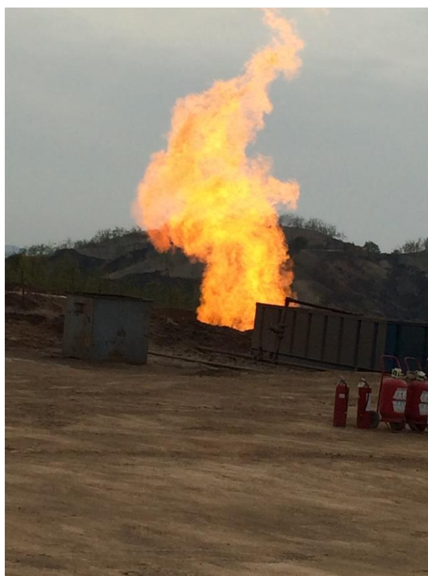
TB-2H flare pit testing on Linxing (West)
