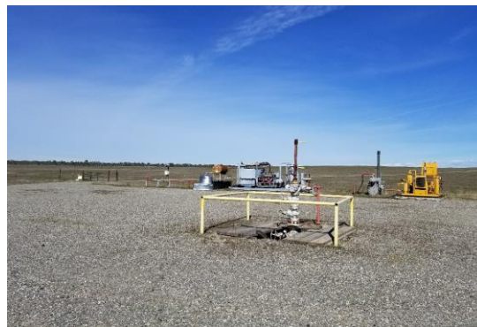
Fig. 5: Sargasco Operated gas producing well
