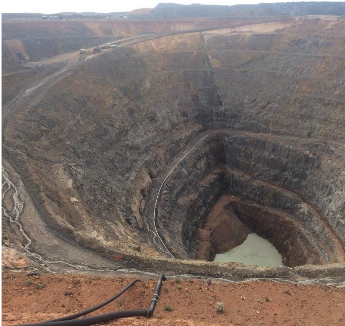
Substantially dewatered Cosmos open-pit at end of June
