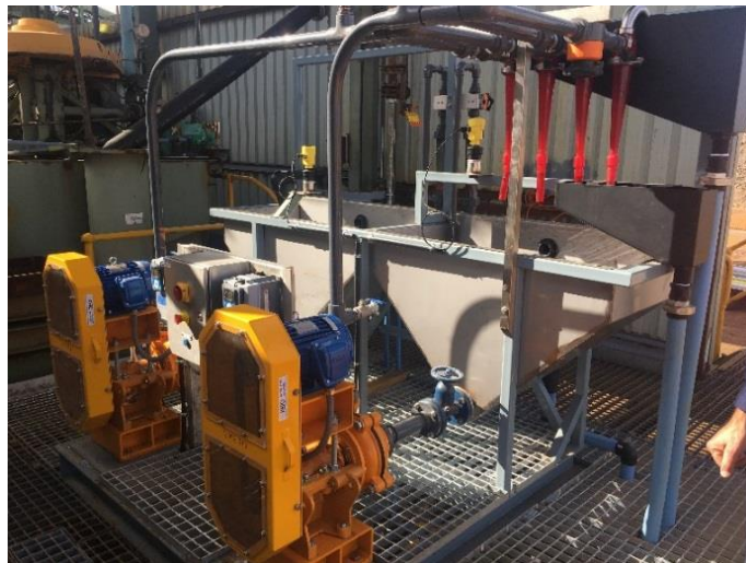
De-slime unit for MREP tailings being installed
