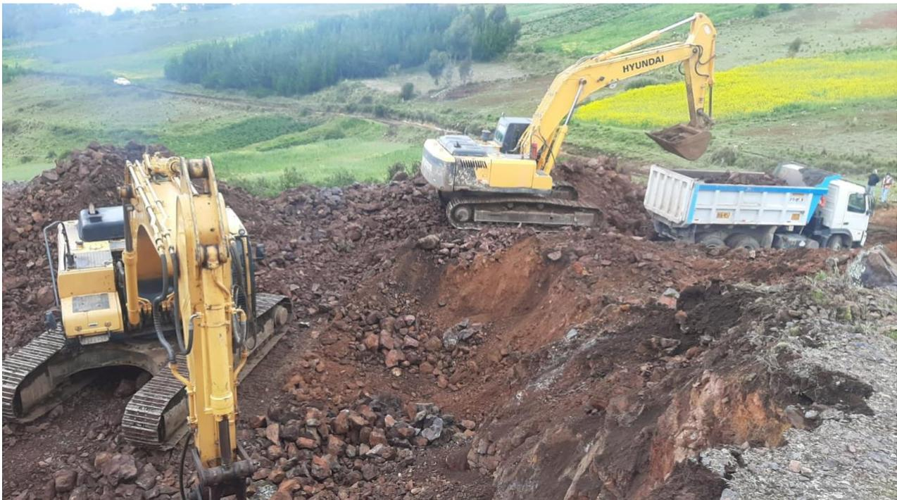
*Figure 2. Loading of Ore onto trucks for delivery to crushing plant*
